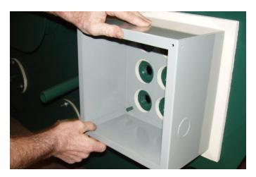
4) With the nuts provided, tighten the box against the gasket until the gasket compresses slightly.
