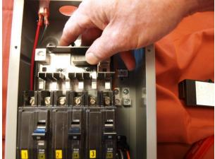
This shows removing the SFBA after loosening the six (6) slotted head, breaker screws. Be aware the screws were factory set quite tight.
