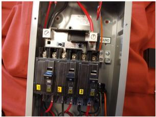
This shows a single 90 amp x 240 vac feed with the plastic safety cover removed. Tighten both main lug screws securely. The plastic cover must be reinstalled before the 90 amp feed circuit is activated. In all cases, follow the NEC for wire sizing. The ground wire is not shown for clarity, but *grounding is required in all cases*.
